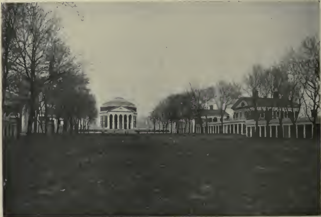
South Front of Rotunda.
